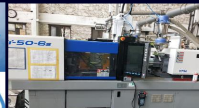
Replacement of hydraulic m/c & pneumatic screw drivers with electrical ones
